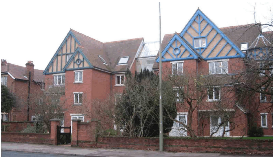
Examples of the erosion of corner plots in the Conservation Area
